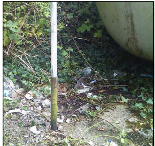
Protected metallic pipework entering the ground
